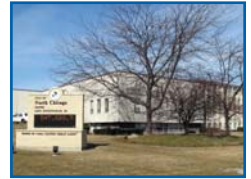
North Chicago Municipal Complex
